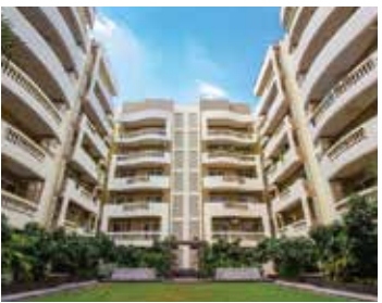
SHALIMAR DWELLING AP SEN ROAD LUCKNOW
