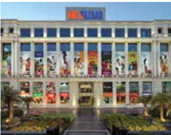
SHALIMAR ELLDEE PLAZA BHOOTNATH MARKET LUCKNOW
