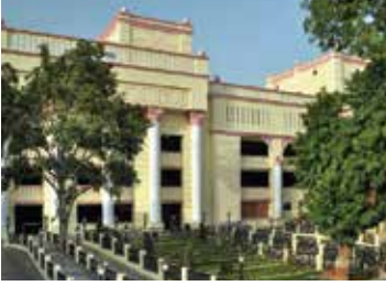
MULTILEVEL PARKING HAZRATGANJ LUCKNOW
