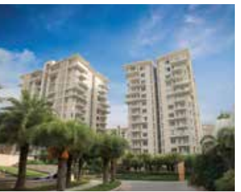
SHALIMAR GALLANT MAHANAGAR LUCKNOW UPRERAPRJ3168
